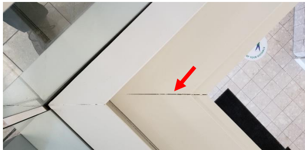
Figure 29. Separations in wood trim at mitered corners adjacent to main stair opening on the second floor
