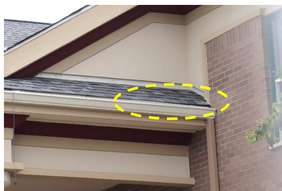
Figure 39. Edge metal and edge of shingles appear out of plane with roof edge.
