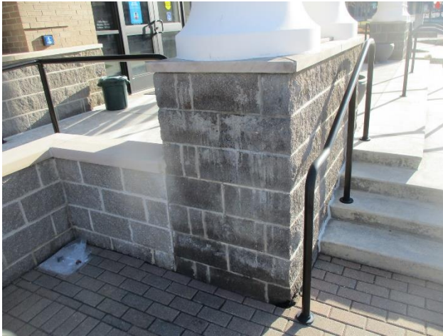
Figure 8. Water staining at the portico column base near the south entrance of the building
