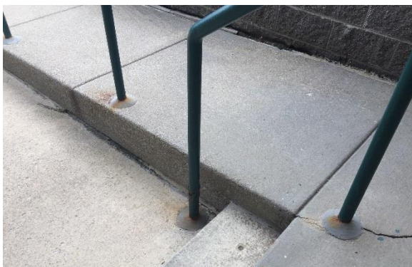
Figure 14. Corrosion and staining at the base of the handrails on the north side of building
