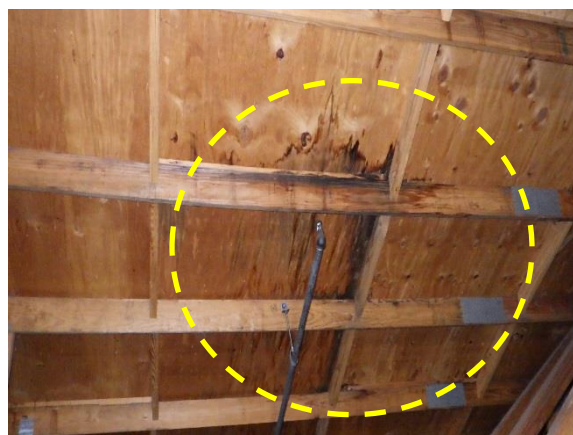
Figure 51. View of deteriorated plywood roof sheathing and 2x framing
