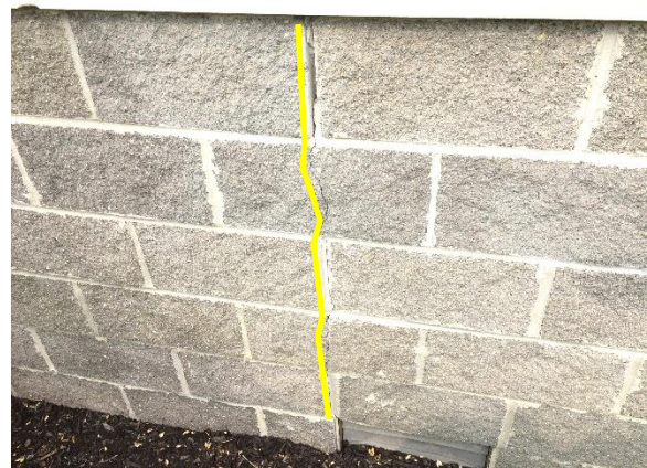
Figure 9. Vertical crack in CMU (shown in yellow)
