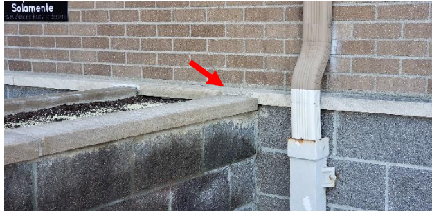
Figure 33. Approximately 3/4-inch of vertical displacement of the planter adjacent to the north exterior building wall
