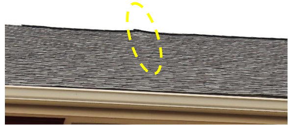
Figure 29. Raised shingles on south face at west gable
