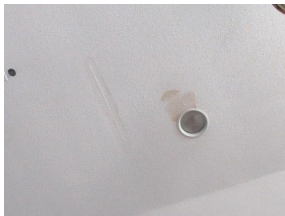
Figure 49. View of water staining on the ceiling
