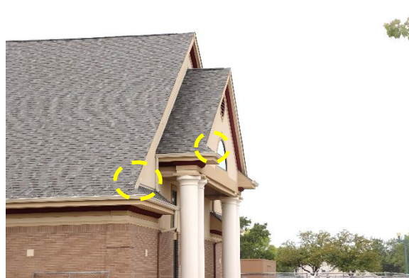
Figure 37. Deterioration of fascia where it meets roofing plane
