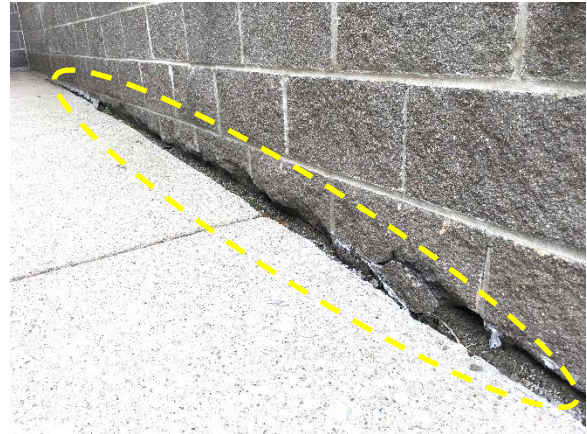
Figure 13. Spalled and cracked CMU along the joint between the wall and concrete ramp
