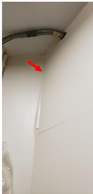
Figure 25. Cracked gypsum sheathing at second floor janitor's closet
