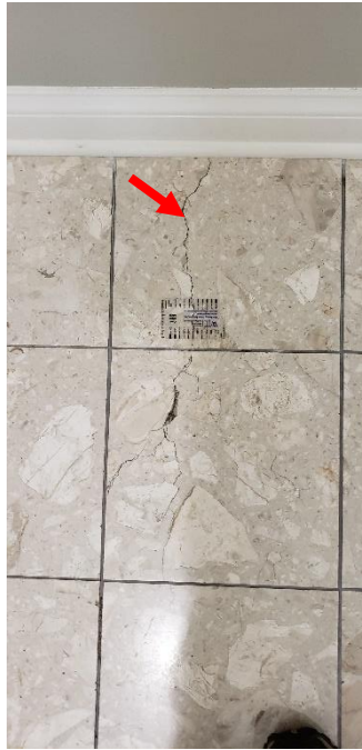
Figure 19. Cracks in floor tiles below landing of main stairway
