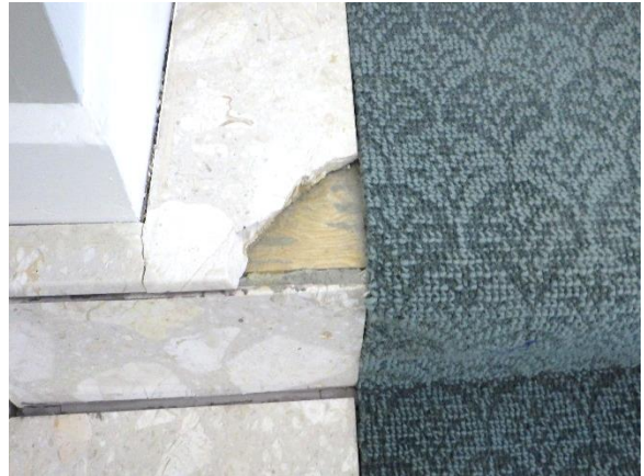
Figure 43. Broken floor tile at entry stairs
