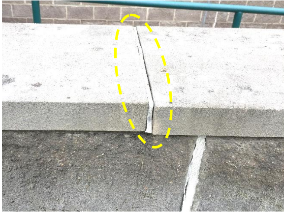
Figure 16. Failed sealant head joint between limestone copings
