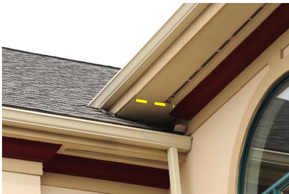
Figure 26. Crack in EIFS soffit
