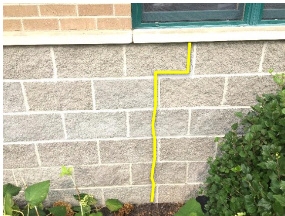
Figure 8. Vertical and stair-stepped cracks in the CMU (shown in yellow)
