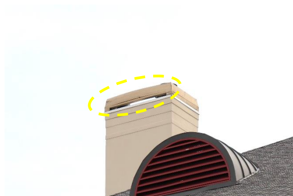
Figure 34. Deterioration of wood on chimney
