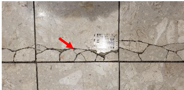
Figure 17. Cracking of floor tile at first floor around elevator and near janitor's closet
