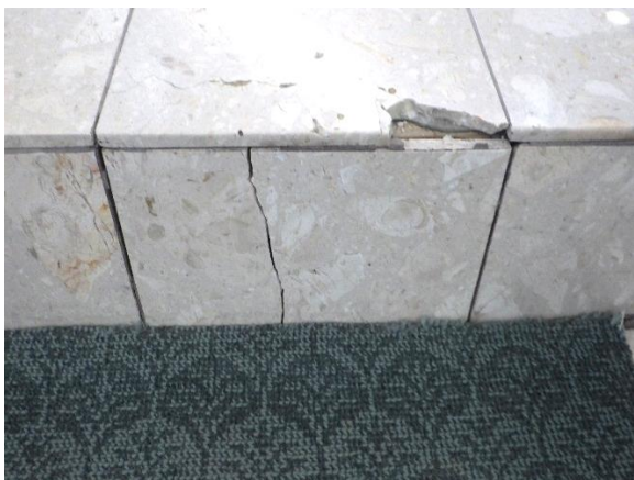
Figure 44. Cracked and broken floor tile at entry stairs
