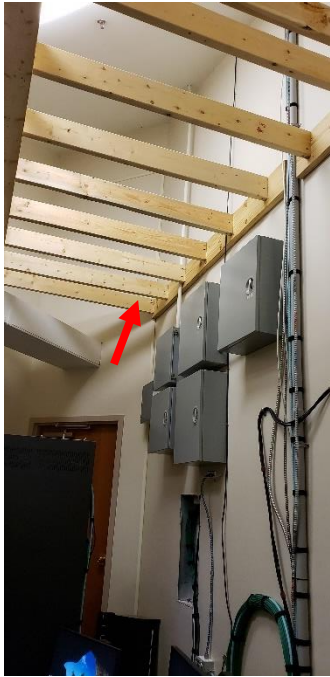
Figure 22. Wood bracing in A-V room at the northwest corner of the Auditorium to support televisions hung from the walls
