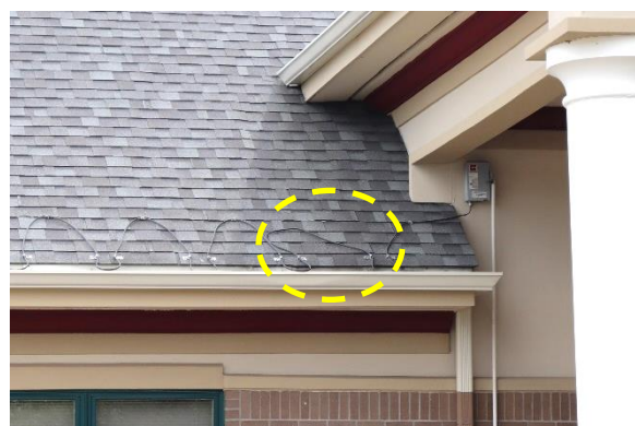
Figure 38. De-icing cable detached from clip
