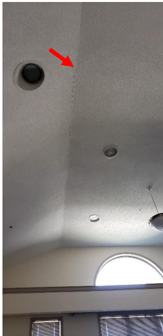
Figure 20. Cracks in gypsum sheathing of Auditorium
