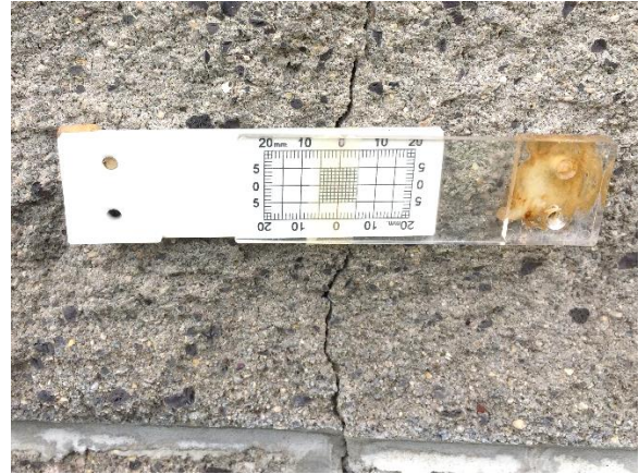
Figure 11. Existing crack monitor on west exterior wall
