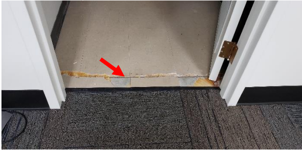
Figure 26. Cracked floor tiles at door threshold to the server room at the second floor
