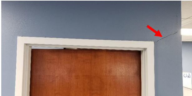
Figure 18. Crack in wall widened at increasing height
