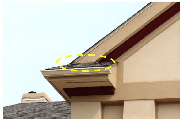
Figure 27. Deterioration of fascia where it meets roofing plane
