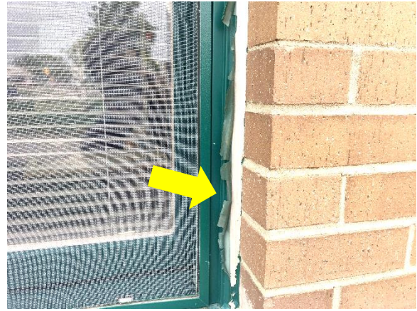
Figure 23. Flaking paint on window frame
