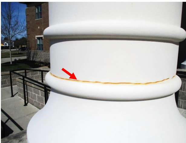
Figure 12. Corrosion staining at the base of the portico column near the south entrance
