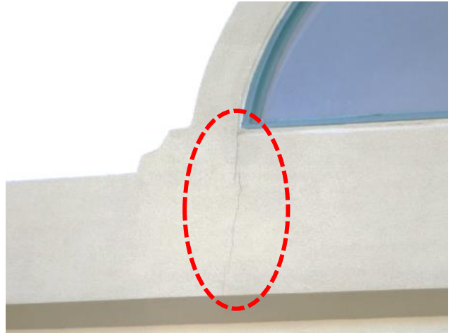
Figure 9. Crack in EIFS lamina at north portico window
