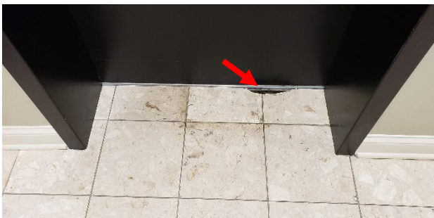
Figure 24. Cracked floor tile in front of elevator at the second floor
