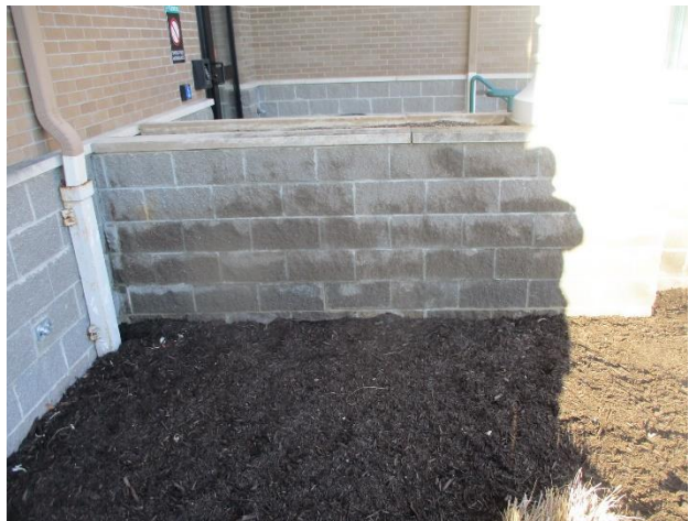
Figure 7. Water staining on the CMU partial wall near the northeast entrance
