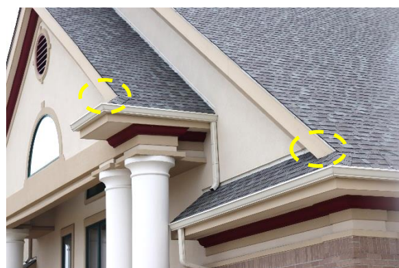
Figure 36. Deterioration of fascia where it meets roofing plane
