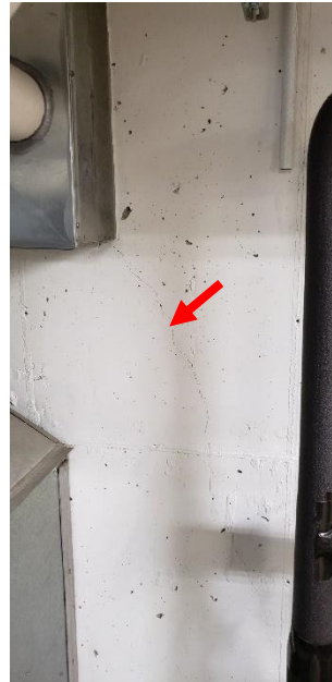
Figure 15. Hairline, vertical cracking on west wall of concrete basement
