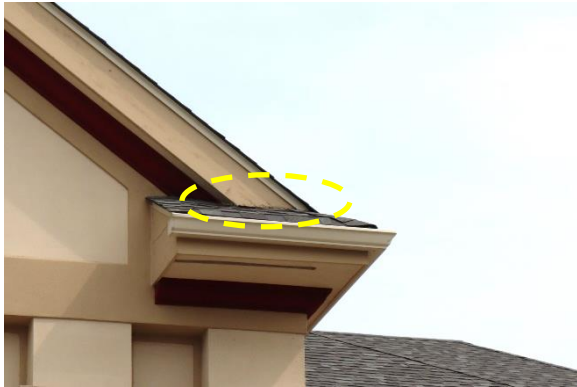
Figure 28. Deterioration of fascia where it meets roofing plane
