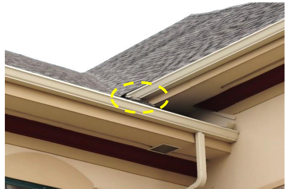
Figure 33. Deterioration of fascia where it meets roofing plane
