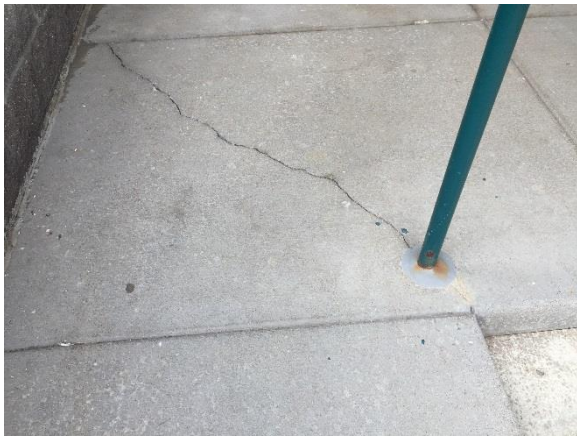
Figure 24. Cracked sidewalk slab on north side of building
