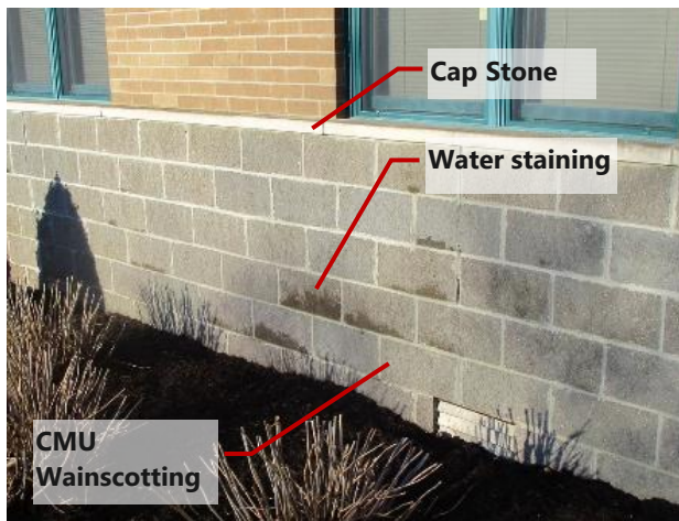
Figure 6. Water staining on split face CMU wainscoting
