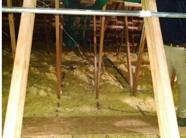
Typical Attic Area Needs Added Insulation.
