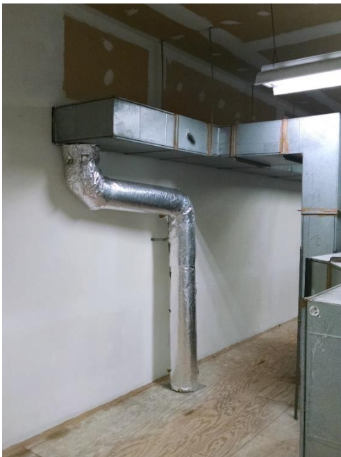
Typical Supply Duct Added for Space Cooling.
