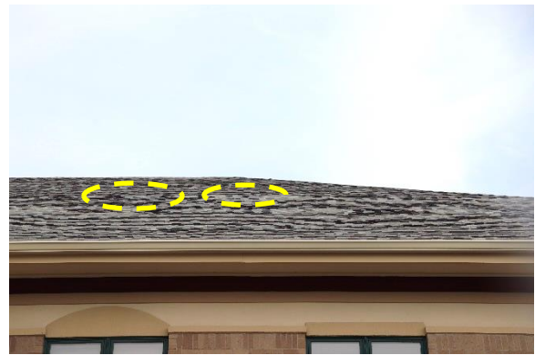
Figure 31. Raised shingles on south face at east gable
