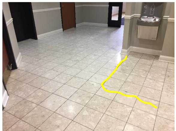
Figure 45. View of cracked ceramic floor tile
