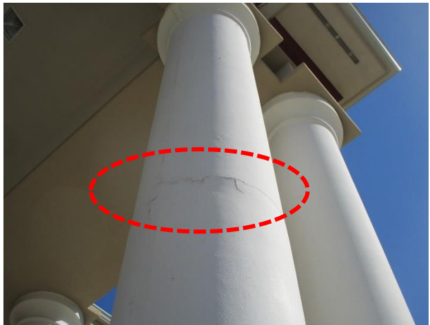
Figure 11. Cracked coating at portico column near the south entrance
