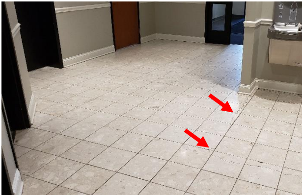
Figure 16. Cracking of floor tile at first floor around elevator and near janitor's closet
