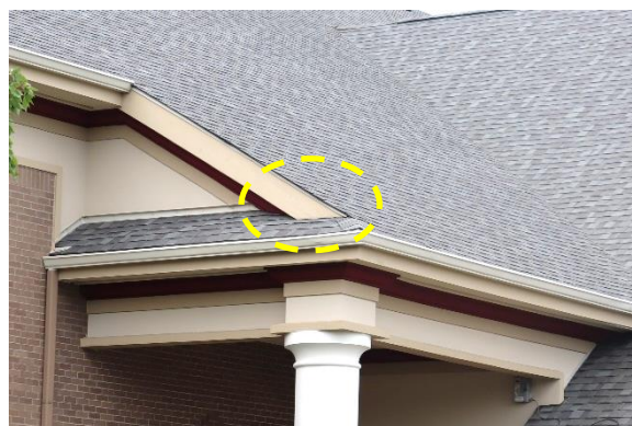
Figure 35. Deterioration of fascia where it meets roofing plane
