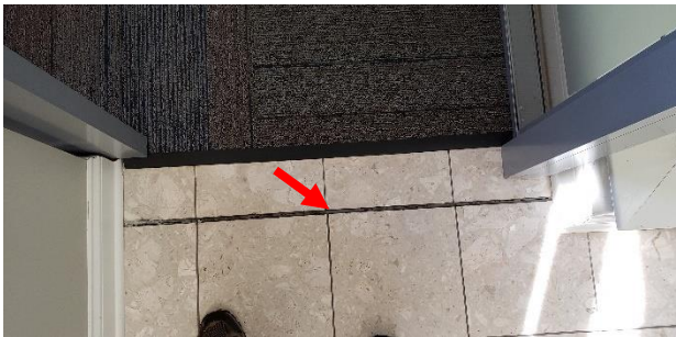
Figure 28. Cracking in joints of floor tiles adjacent to main stair opening on second floor
