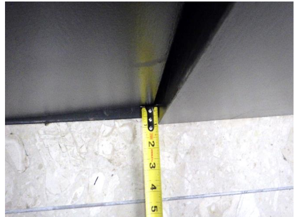
Figure 55. View of misalignment of doors in the closed position at the auditorium
