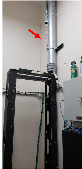
Figure 27. Crack in gypsum sheathing at northeast corner of server room on second floor
