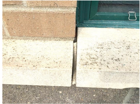
Figure 17. Cracked and missing mortar at a head joint between limestone accents
