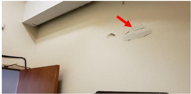
Figure 23. Tearing of gypsum sheathing finish in A-V room of the Auditorium
