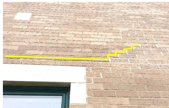
Figure 21. Cracked mortar joint (shown in yellow)
