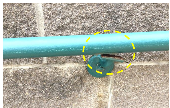
Figure 15. Broken handrail connection
