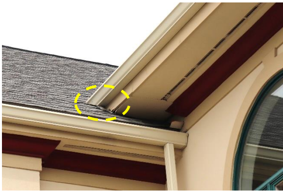
Figure 30. Water damage of fascia at roofing plane
