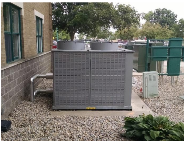
Air Cooled Chiller Replaced in 2017.
