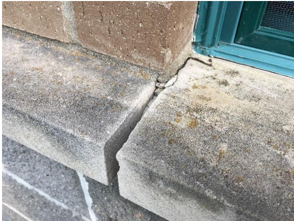
Figure 18. Missing mortar at head joint between limestone accents
