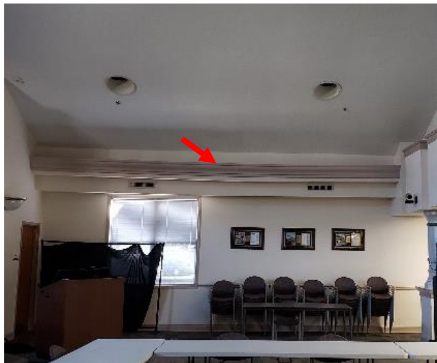
Figure 21. Sagging of duct on east wall of Auditorium
