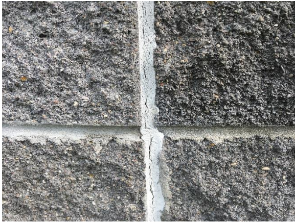
Figure 22. Cracking sealant at expansion joint
