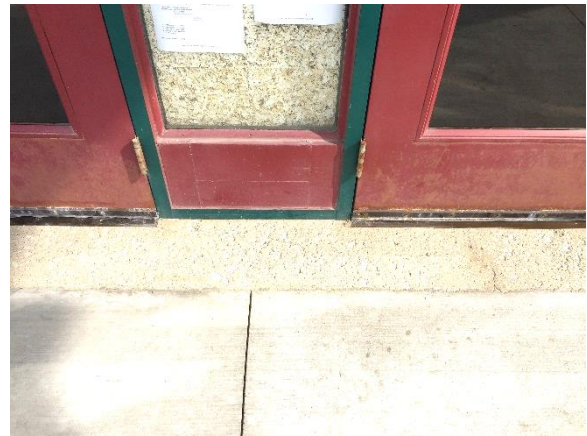
Figure 25. Corrosion and rust staining visible at base of main entry doors
