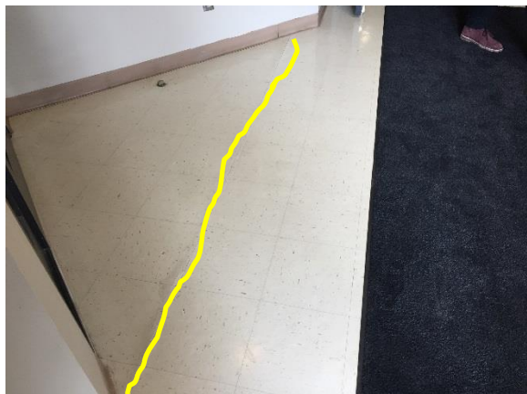
Figure 46. View of cracked vinyl floor tiles
