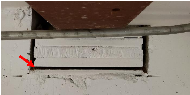
Figure 14. Steel wide-flange beam with gap between the bearing surface of the pocket
