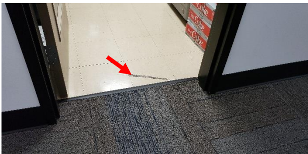
Figure 30. Cracked tile in administration office kitchenette
